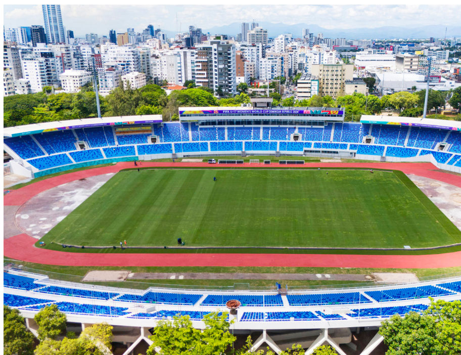
The Organizing Committee is focused on the adaptation and modernization of the sports facilities.
