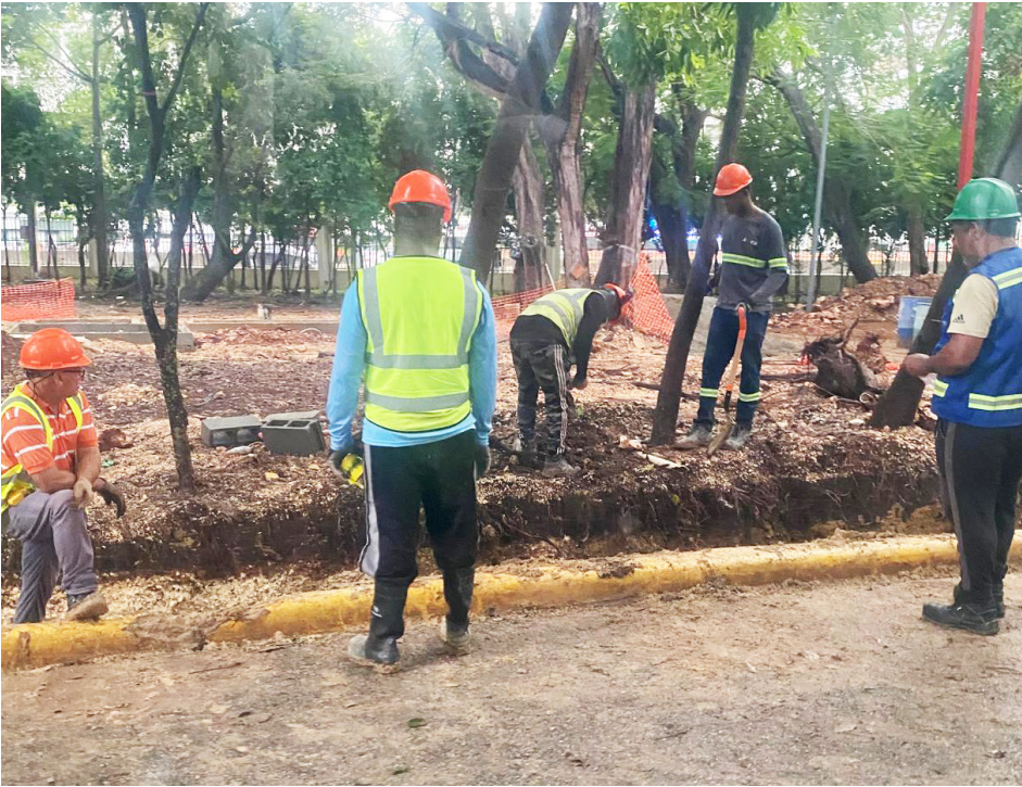
Workers are working on the remodeling and construction in different areas of the Olympic Center.
