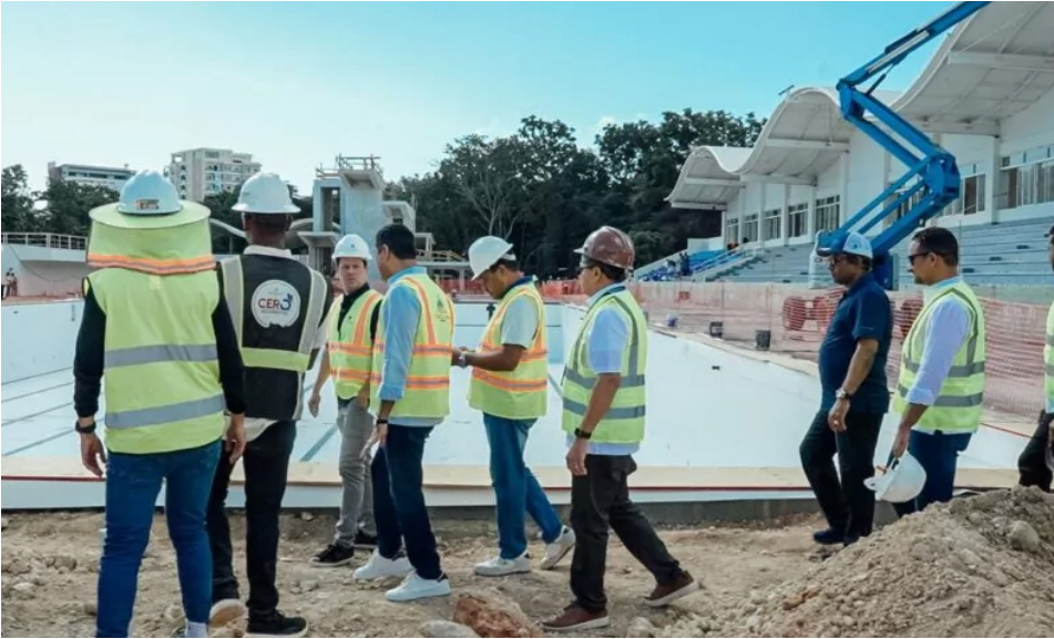
Technicians and authorities oversee the final phase of construction at the Juan Pablo Duarte Olympic Center.
